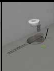
CUTTING A HOLE FOR THE WASTE FITTING
