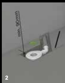
CUTTING A HOLE FOR THE WASTE FITTING
